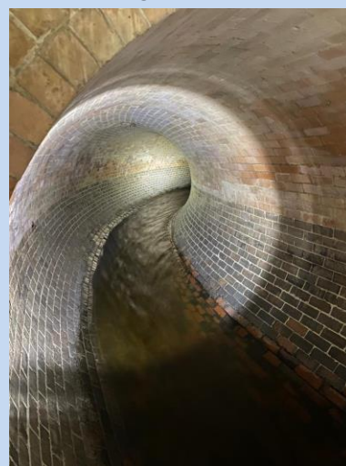
Photo 2.2: The Platteklouf River, which is passed under the City Bowl in covered, brick-lined culverts
