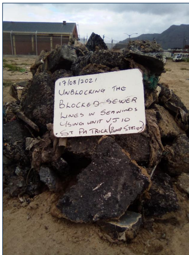
Photo 7.1 Rubble and other waste dumped in sewers contributes to blockages and overflows Photo courtesy CCT (Mr A. Taylor)
